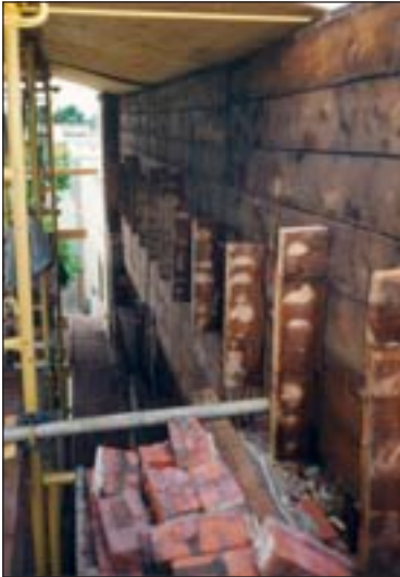
This building's brick veneer was removed to expose and repair rot occurring in the underlying wood frame construction.
