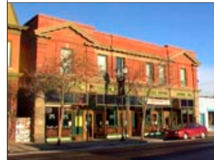
Masonry piers link the Carson Block's upper and lower facades and define bays at either end of the building (see below). But the piers' transition from sandstone to brick also serves to keep the building's upper and lower levels distinct.
