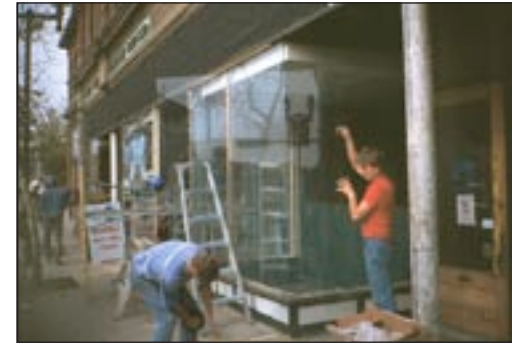
Installation of plate glass windows on the Carson Block.
