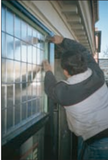
A local glass craftsman repaired the original leaded glass clerestory windows of the Fraser Block, retaining as much historic fabric as possible.
