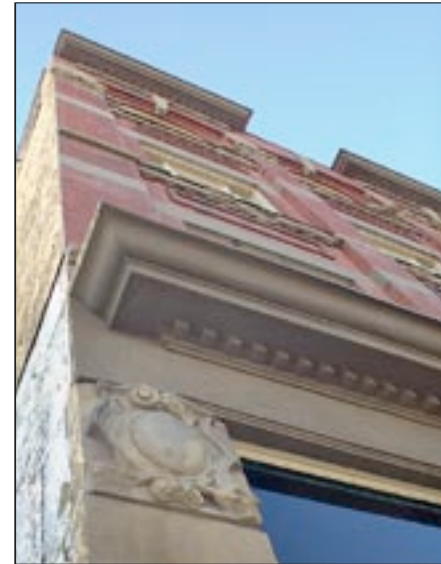
The lower cornice of the Fraser and Seabloom Block features a distinctive moulding profile, decorative “dentils,” and a sand-paint finish. The continuous lower cornice balances this building’s unusual split upper cornice.
