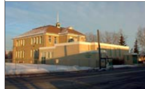
The Alexandra Centre represents several, radically different, phases of masonry construction. The original school at the rear of the complex, distinguished by its quarry-faced sandstone exterior, is obscured by much later, post-World War II concrete block addition nearest the street.
