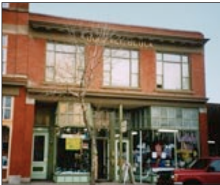
Photographs of the Dougall Block before and after facade rehabilitation illustrate the impact of exposing and reinstating the clerestory windows. The display and upper floor windows have also been restored to their original dimensions.
