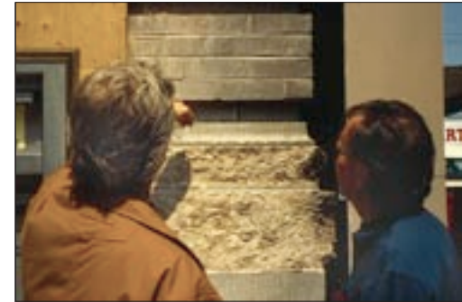
Architects inspect original brick and Tyndall stone details beneath a “slip cover” on the CIBC building as part of preliminary planning for the building rehabilitation project. The stone details had been hacked away by renovators and were costly to replace.
