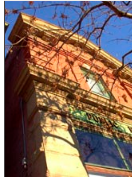
Masonry piers link the Carson Block's upper and lower facades and define bays at either end of the building (see below). But the piers' transition from sandstone to brick also serves to keep the building's upper and lower levels distinct.
