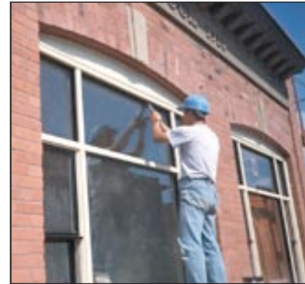
The upper windows on the Befus Block are restored to their original size and configuration with high-performance thermal pane units. The bracketed cornice detailing is visible above.
