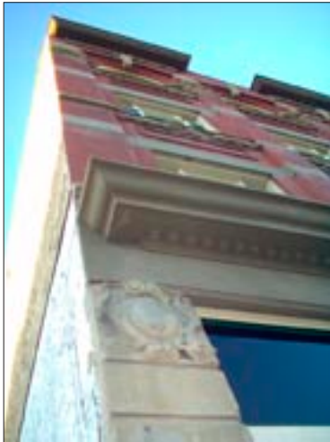
The masonry and sandstone elements of the Fraser and Seabloom Block underwent an extensive cleaning program.
