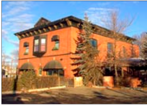
The elaborate cornice of Fire Station No. 3 is an excellent example of the prefabricated and customized pressed metal facade elements popular in the early 1900s.
