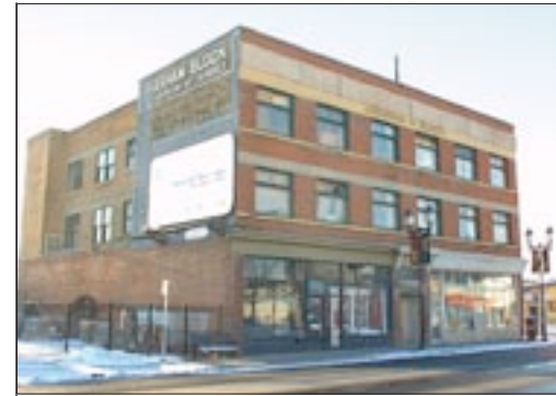
The Gresham Block's large scale, extensive glazed storefronts and broad upper window openings are made possible by structural steel supports and are characteristic of Late Commercial buildings.
