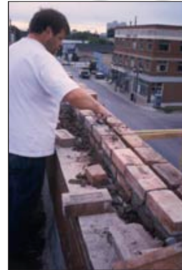
The original parapet wall on the Carson Block was dismantled, repairs were made, and the wall was reconstructed using the original bricks.
