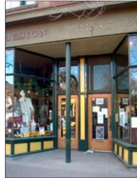
A steel column helps support the wide recessed entrance needed for these twin doorways on the Burn Block.
