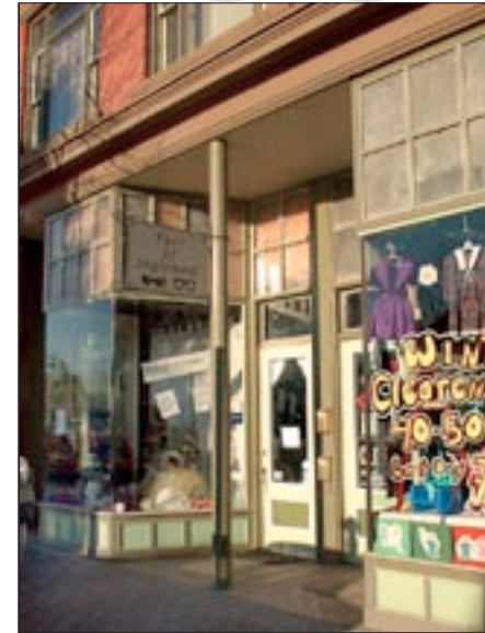
The alignment and detailing of bulkhead panels on the Dougall Block match the rhythm of the clerestory windows above, lending continuity to the outward-facing and recessed portions of the storefront and drawing the pedestrian's eye inward from the sidewalk.
