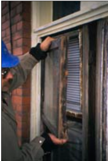
Individual storm windows are removed from the Fraser Block for restoration.
