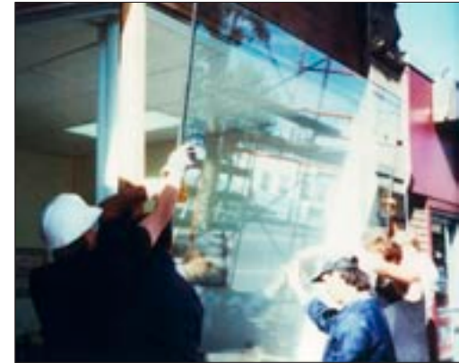
Installation of new display window glass in the Fraser and Seabloom Block.
